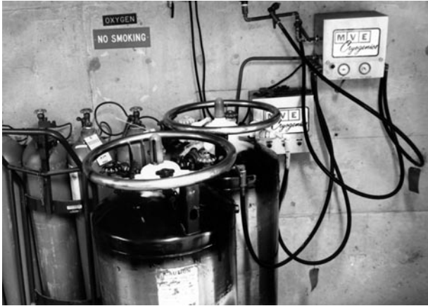
Figure 16-6. Liquid oxygen cylinder delivery system. Note the reserve supply of oxygen cylinders connected to a manifold for a back-up system.
