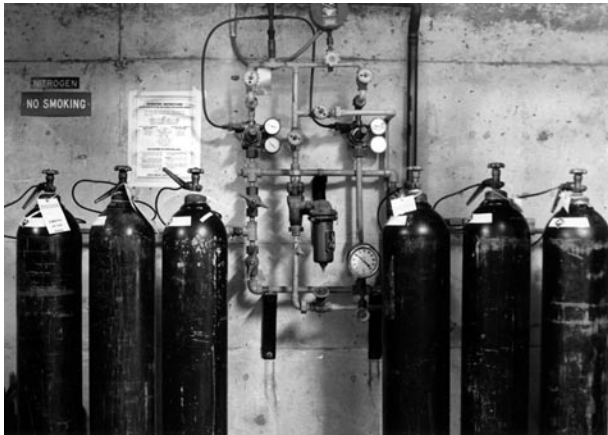
Figure 16-4. Manifold for connection of several compressed gas cylinders to a pressure regulator and common gas line. This is a system for delivery of nitrogen.
