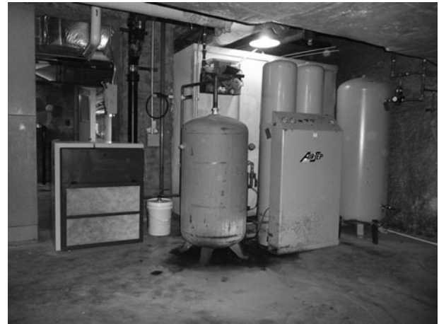
Figure 16-5. This oxygen generator is capable of producing 22L/min of oxygen. (Air Sep Corp, Buffalo, NY.)
